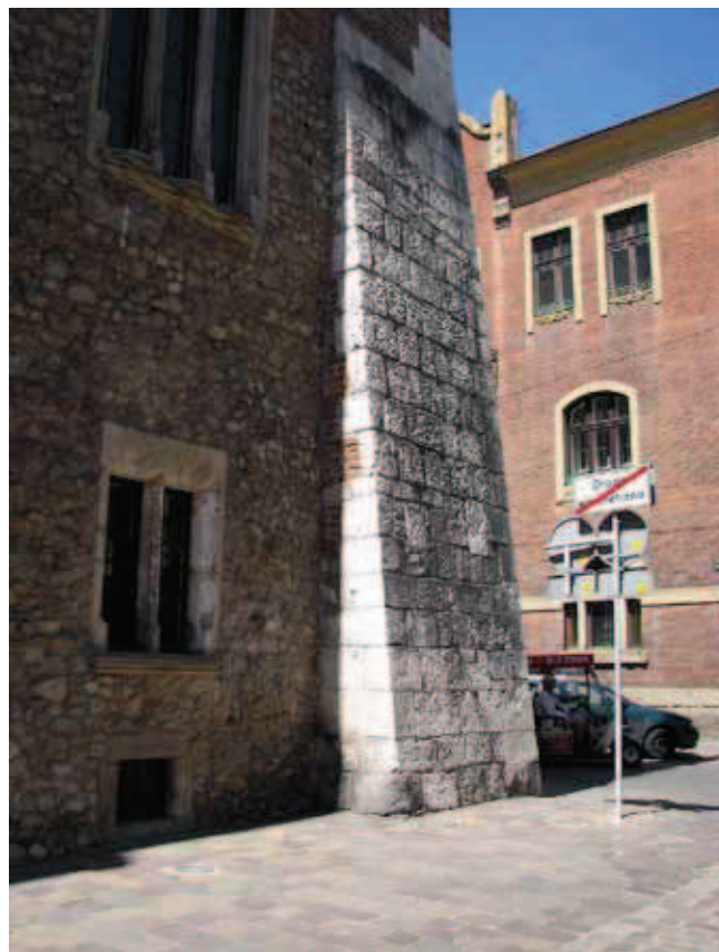
Fig. 8. Collegium Maius building with escarpment made of the Upper Jurassic grand appareil blocks, as well as fragments of the opus incertum wall made of the same material, phot. A. Majer-Durman • Budynek Collegium Maius na rogu ulic Jagiellońskiej i św. Anny. Widoczna skarpa z bloków grand appareil z wapienia górnojurajskiego oraz fragment muru opus incertum z tego surowca, fot. A. Majer-Durman
