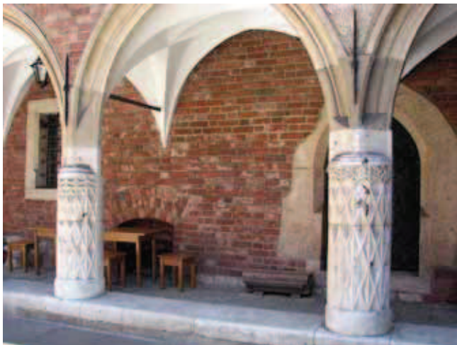
Fig. 10. Columns made of massive limestone with flints in the courtyard of the Collegium Maius, phot. A. Majer-Durman • Kolumny wykonane z wapienia skalistego z krzemieniami na dziedzińcu Collegium Maius, fot. A. Majer-Durman
