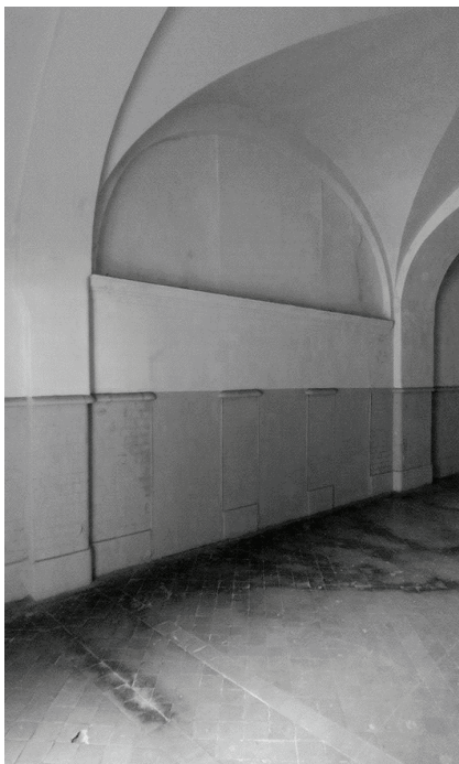
Fig. 7. Opole Station East – bricked up window [Photo taken by authors].
