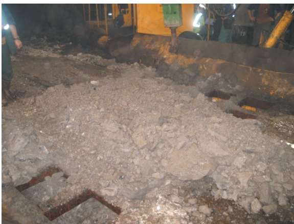
Fig. 4. Grate after LKP-0903 loader has unloaded excavated material
