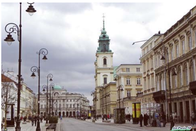
Fig. 6. Fragment of the Royal Route, Krakowskie Przedmieście street – view at Staszic Palace after refurbishment of this street in the beginning of 21st century. Source: [21]
