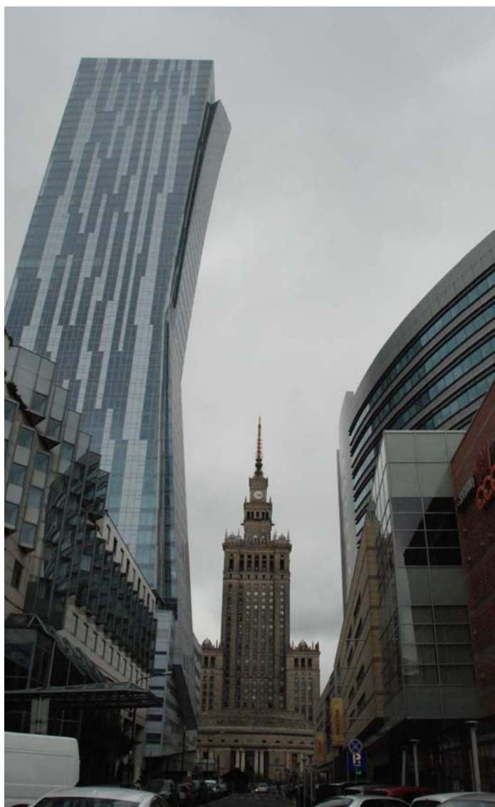
Fig 26. A view from the west to the Palace of Culture and Sciences. On the left, a building designed by Liebeskind, with a swinging, dynamic, postmodernist form and (presumably) untypical front panelling. On the right, a soft form of "Złote Tarasy" shopping centre. Source: picture by K. Guranowska-Gruszecka 2016
