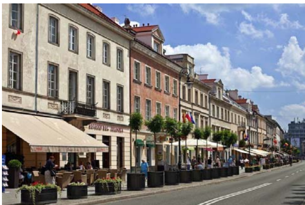
Fig. 5. Fragment of the Royal Route, Nowy Świat street – after reconstruction in classical style. Source: [6, p. 135]
