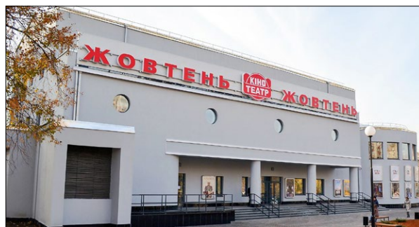
Fig. 3. Zhovten Cinema in Kyiv after the restoration, 2015; photo by https://uk.wikipedia.org/ .
