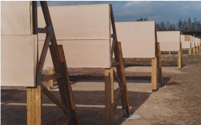
Picture 2. Additional vertical screens placed one after the other, intended to capture ricochets from technical elements and targets in the shooting zone
