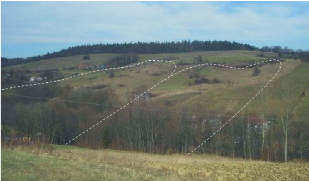
Fig. 2. General view of the “Bystrzyca” landslide
