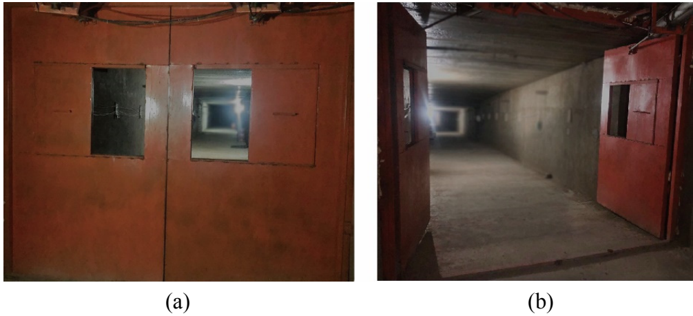
Fig. 4. Field experiment of mine air door
