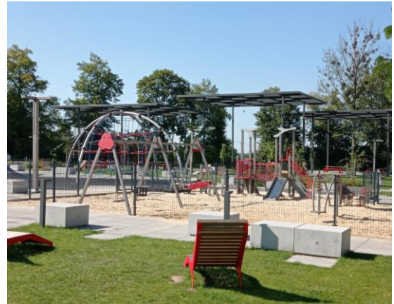
Fig. 2. Revitalised Historic Public Space, Historic Ignacy Mine in Rybnik. Source: Anna Stefańska
