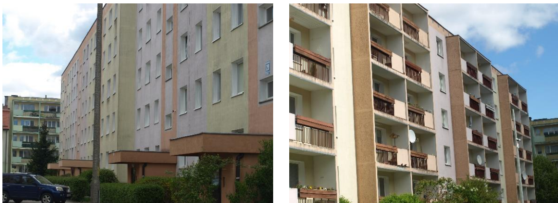
3. Fig. 2. Residential building of the Wk-70 large-panel system - V floor, elevation view: a) north, b) south on the left (Bieranowski P. 2018)
