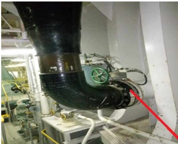
Figure 2. Forward SO x EGCS overboard pipe.
