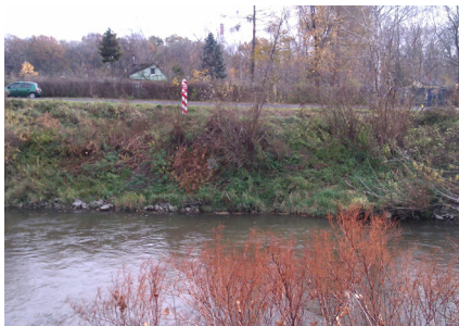
Fig 16. Limited vegetation near urban area – Nysa Łużycka (km 149+300).
