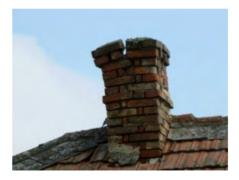
Fig. 13. Destruction of chimney body [source: the Internet]
