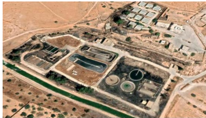
Figure 3. An aerial photo of the wastewater treatment plant in Gharyan city. Source: https://earth.google.com/web/search/32.15153203,13.03476738,662.53720067a
