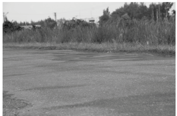
Fig. 6. View of unevenness of the pavement [Own photograph].
