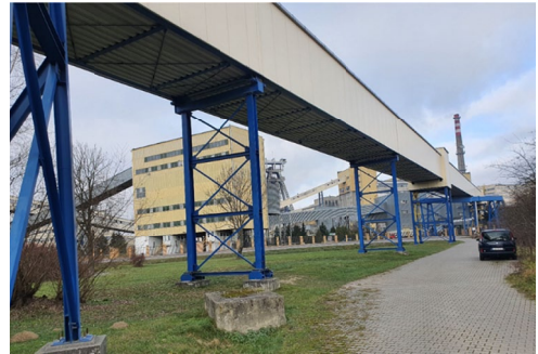
Fig. 3. View of the segment near the industrial plant (300 m) from the south side
