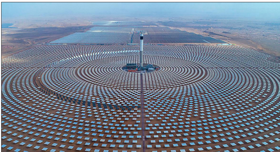
Figure 1. World's largest concentrated solar power plant, Noor Ouarzazate Solar Complex, Morocco (Anouar, 2022)
