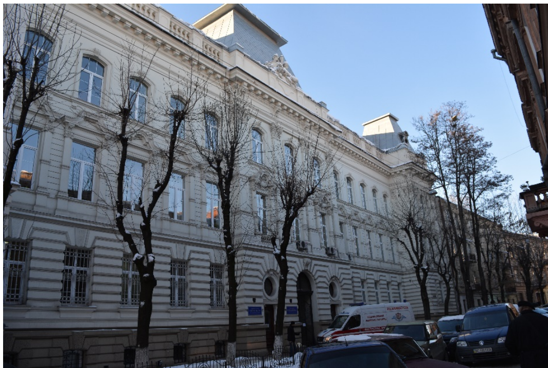
Fig. 8. Building of Railways Directorate and Civil Court (5 Ohienka St.), M. Łużecki, 1895-1897. Source: photo by author (2016)
