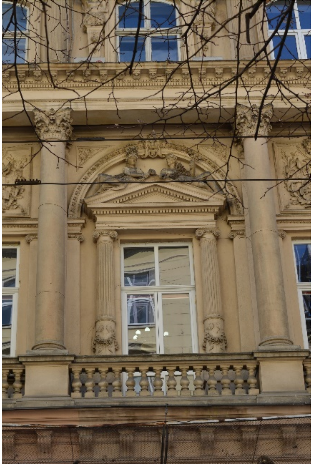
Fig. 4. Railways Directorate. Second storey window of the central façade. Source: photo by author (2016)
