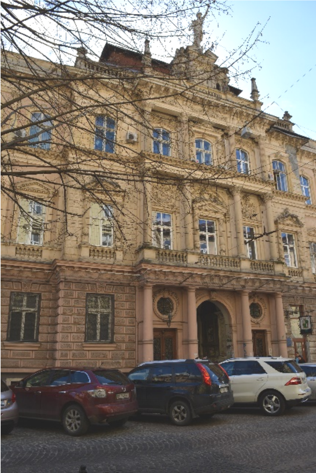
Fig. 3. Railways Directorate (3 Sichovykh Street), architect W. Rawski Junior, 1885-1887. Source: photo by author (2016)
