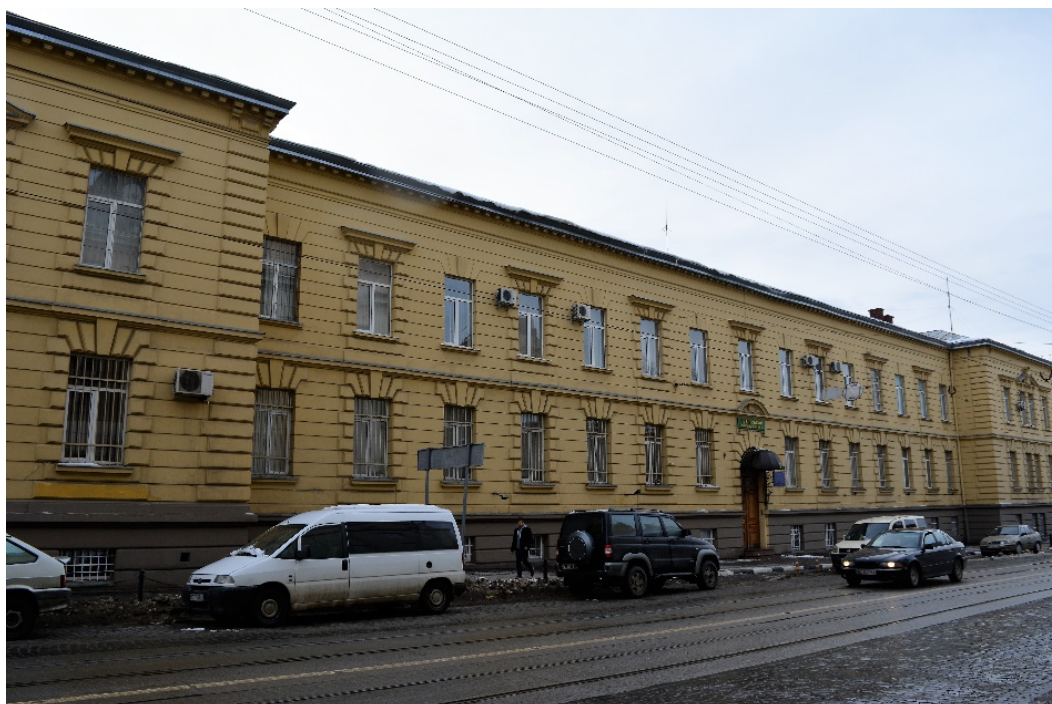
Fig. 9. Military barracks (74 Lychakivska St.). Source: photo by author (2016)
