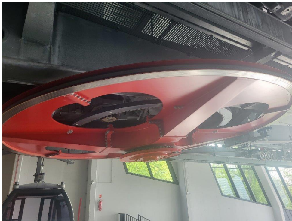
Fig. 7. Jawor station. Platform. Main drive pulley [43]
