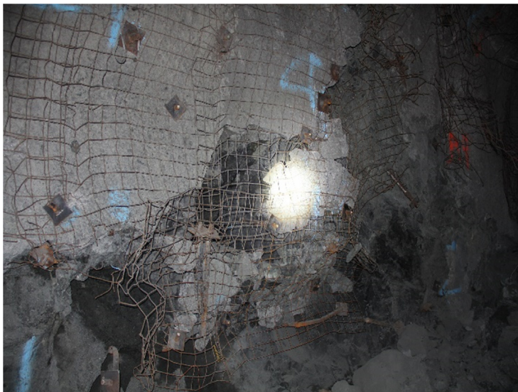
Fig. 6. A rockburst case at diamond mine
