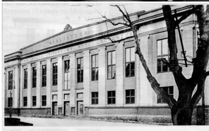
Fig. 2. Building of Research Library Lviv Polytechnic National University. The author professor V. Minkevych. Source: Architecture of Lviv, time and styles XIII-XXI ст., „Tsentr europy”, 2008, Lviv, 540 p.
