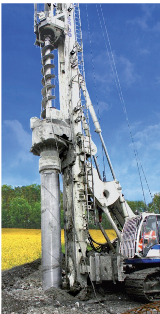
Figure 15. Drilling rig for execution of the pile system CSP
