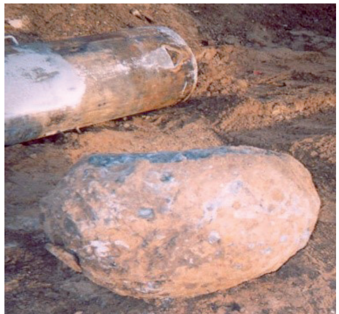
Figure 12. the cases-punch with butt plugged end and excavated rammed pedestal under the pile toe
