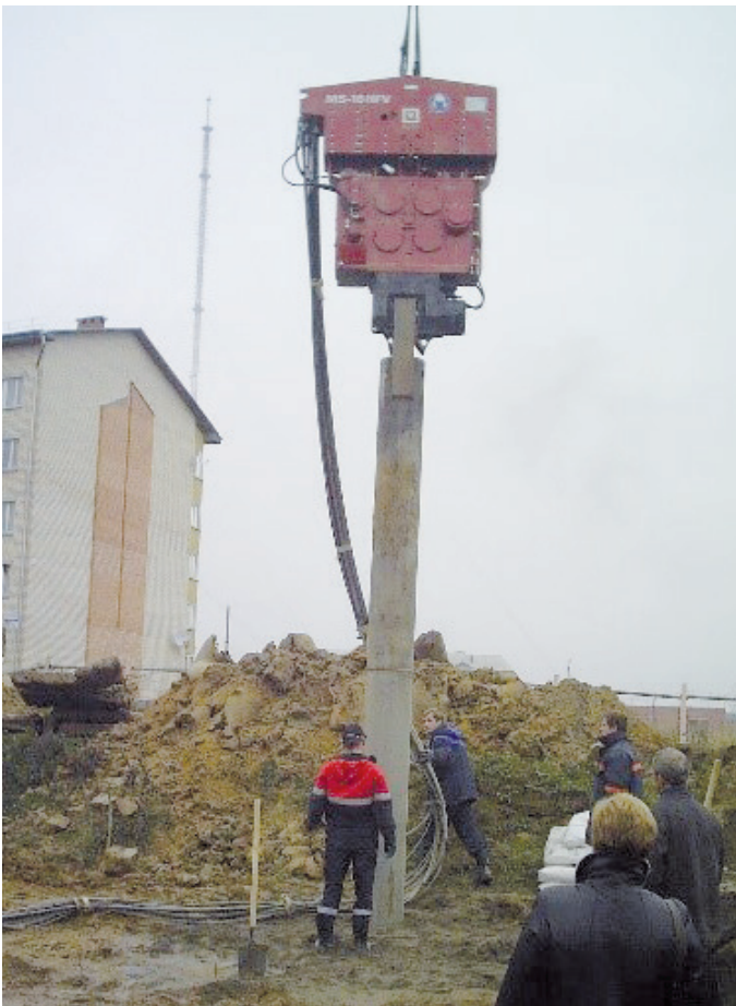
Figure 11. driving tapered casing by using hanging vibro hammer
