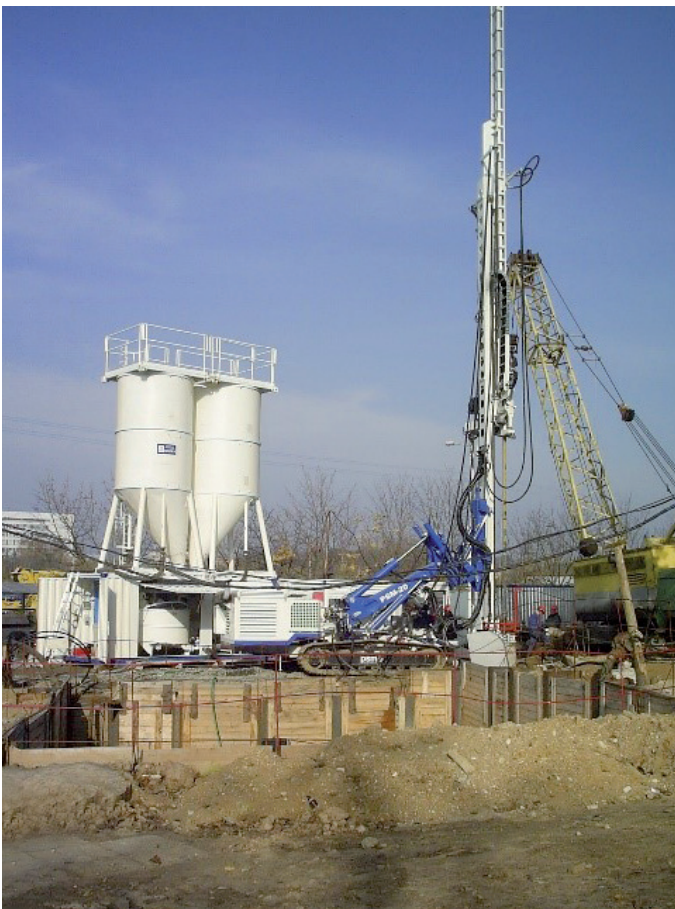
Figure 18. The equipment of Italian company Soilmec for inject technology
