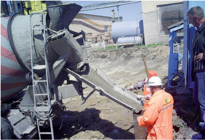
Figure 10. concreting of the casing shaft by mixer
