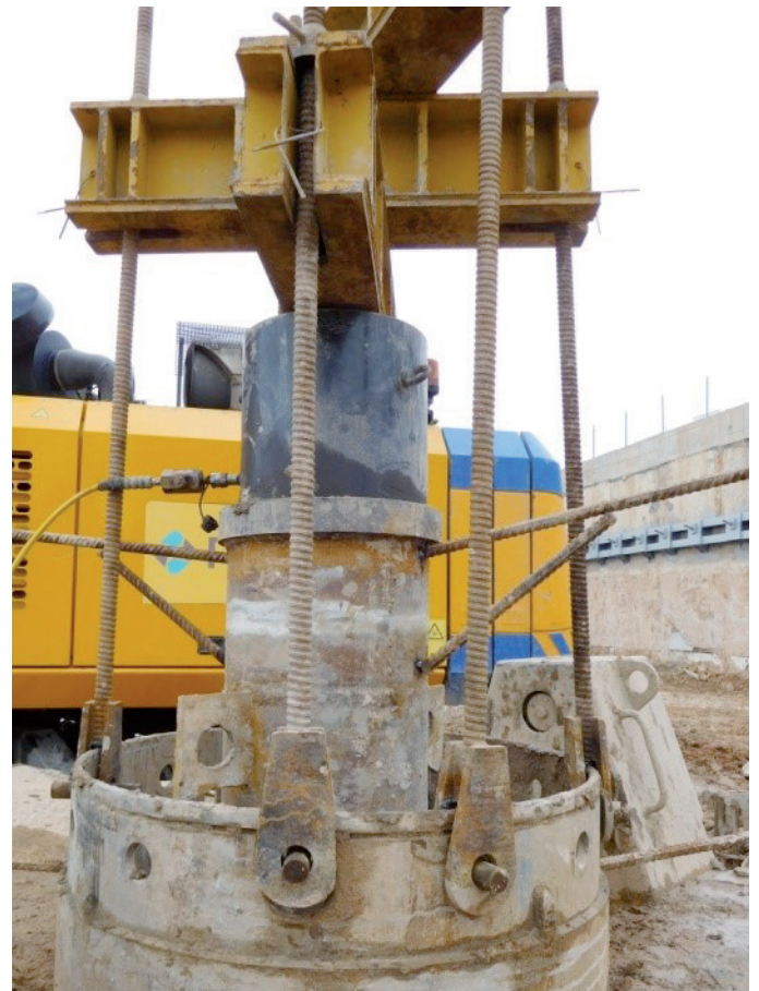
Figure 19. Testing of piles on the principle of «pipe in a pipe»
