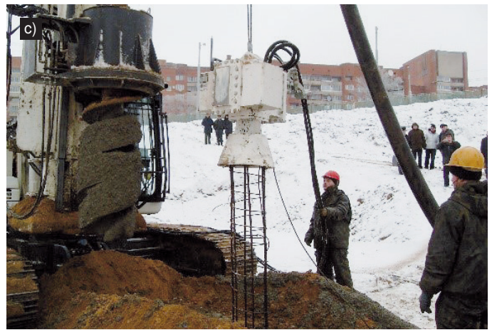
Figure 14. Equipment for piling CFA: a – drilling rig with a solid hollow auger, b – drilling rig for excavating of wells; c – lifting of the auger and installation with the vibro hammer after that installation the reinforcement cage
