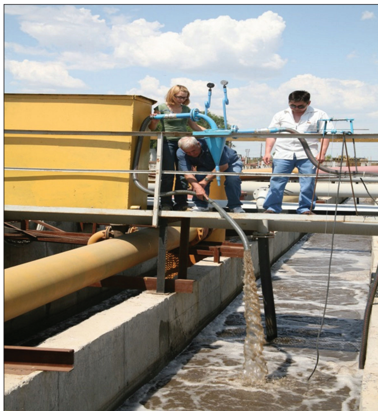
Figure 2. General view of the hydrocyclone-membrane unit
