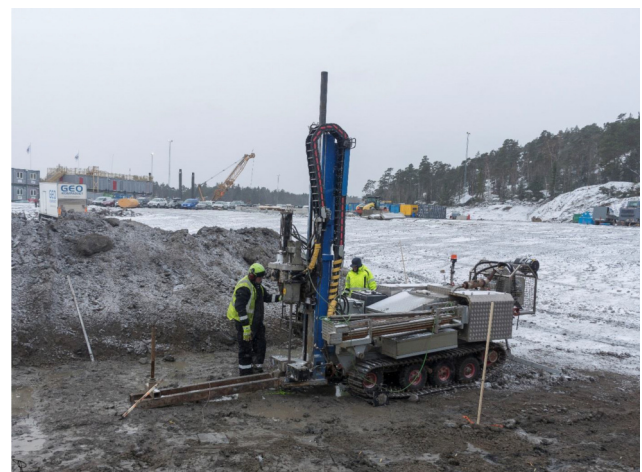
Fig. 1. Process of CPT sounding in Norvik area. Photo source: Per Lindh.
