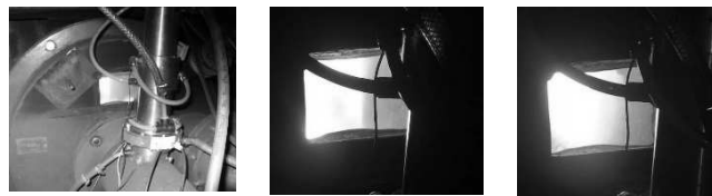
Fig. 4. Plasma pulverized-fuel burner during combustion of coal dust-air mixture [34]
