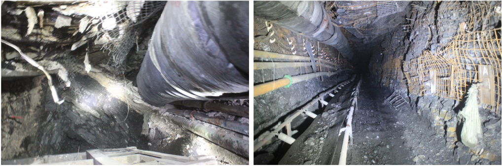
(a) Section without fracturing
