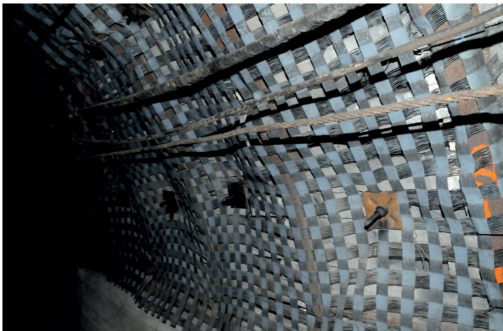
Pic. 2. Constrictive netting Pollux put in the mine workings
