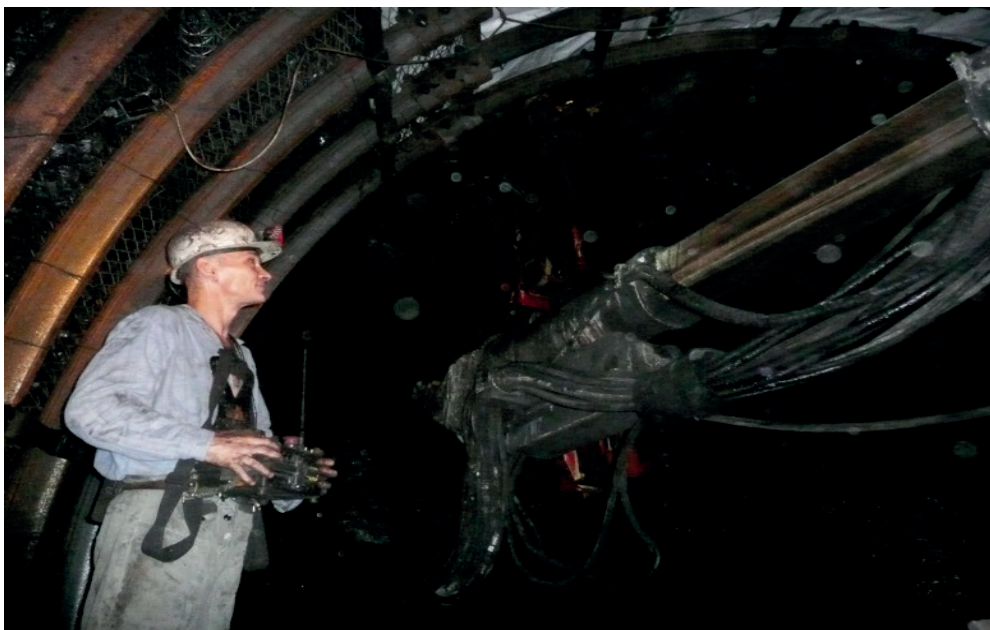
Pic. 1. Remote control of the anchoring process
