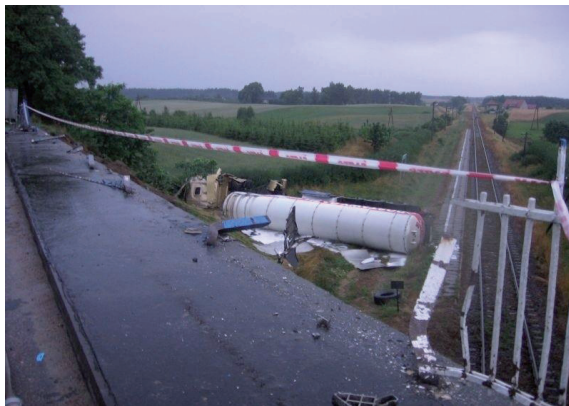
Fig. 1. A 20-tonne tanker fallen from the viaduct over the railroad (line #201) at the stop of Podleś. The tanker transported propane-butane gas [8]
