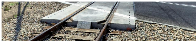
Fig. 8. Concrete level crossing slabs
