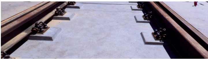
Fig. 7. Module of the level crossing during construction
