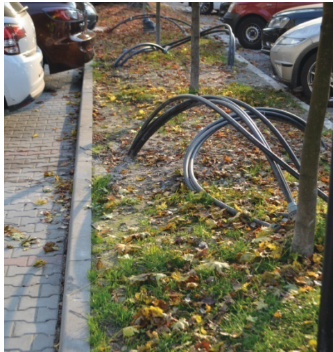
Fig. 2. New research area with oblique borehole heat built in the AGH University of Science and Technology (2017)
