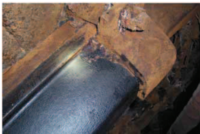
Rys. 6. Obudowa pokryta inhibitorem Fig. 6. Support covered with inhibitor
