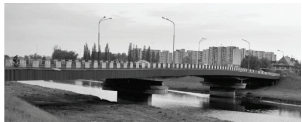
Fig. 1. Niemodliński Bridge, crossed by 20,000 cars per day (photo taken by the authors).
