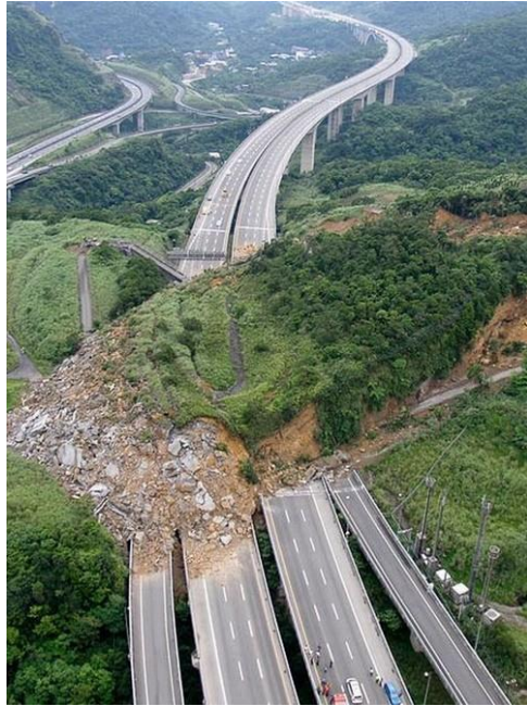
Figure 5. Closed highway due to landslide in Norway in June 2016.
