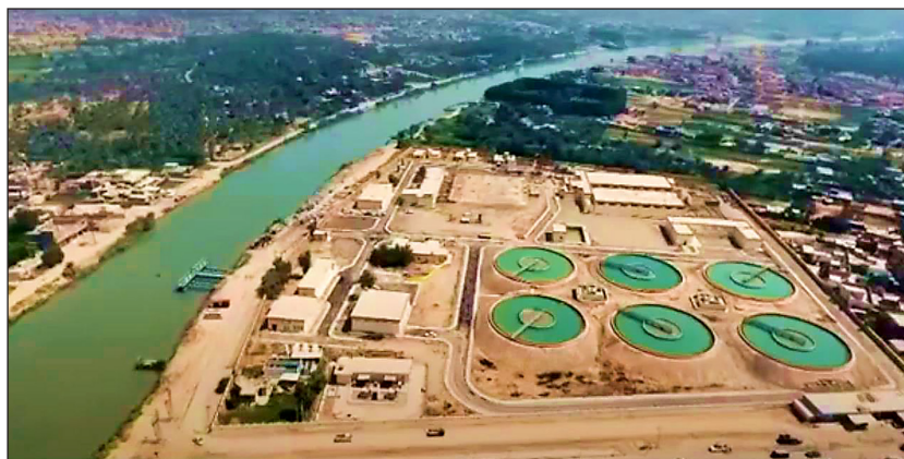
Figure 1. Al-Hashimiyah water treatment plant overview
