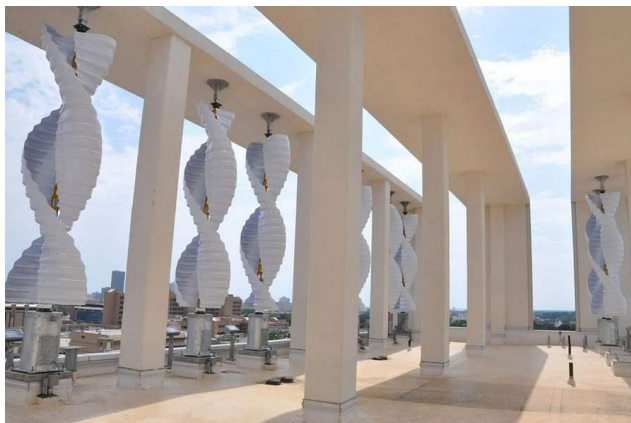
Rys. 8. Turbina Savoniusa [21]
