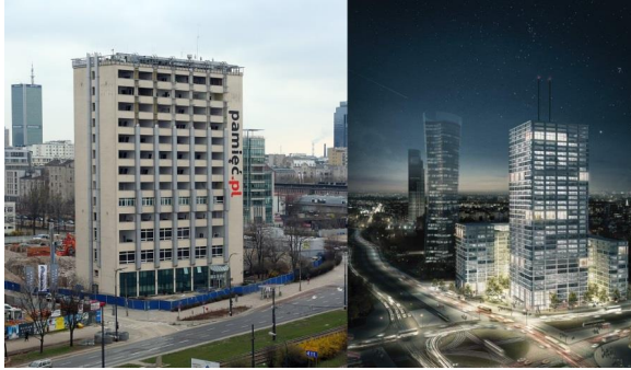
Fig. 5. Photo of IPN's Building for a while before demolition and visualization of Generation Park [Source: [17,19]
