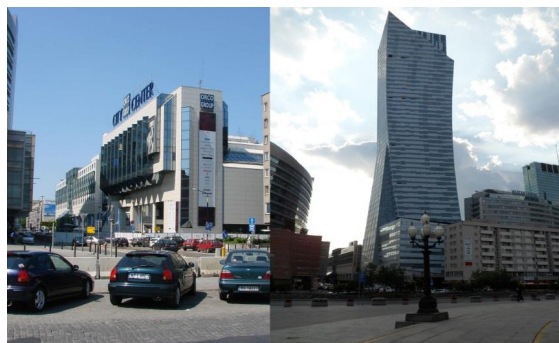
Fig. 4. Photos of City Center and Złota 44
