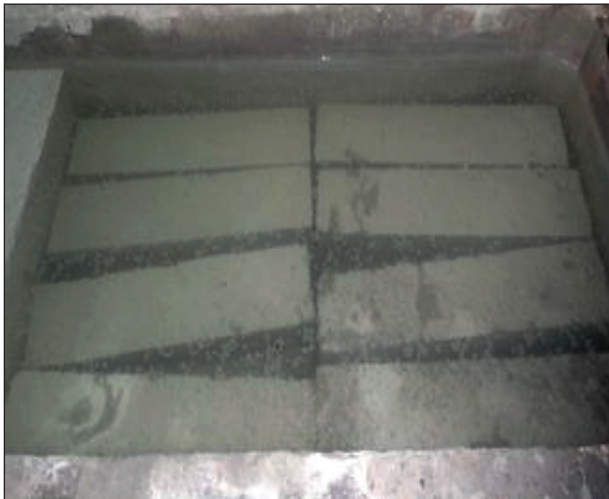
Fig. 4. GR-1 and 4 RC beams curing
