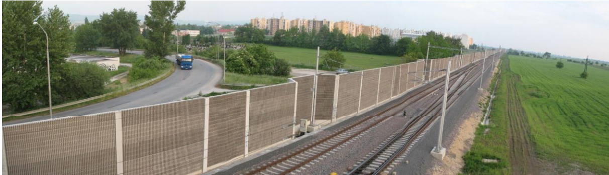
Fig. 15. View of the noise barrier
