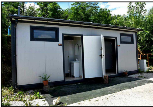
Fig. 4 Container with sanitary facilities. Source: photograph provided by the owner of CNP (by Jolanta Dereszewska).
