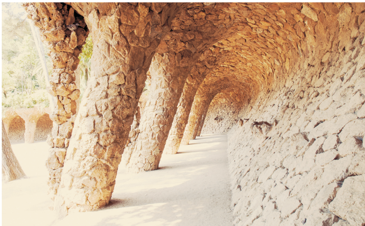
Ryc. 4. Pochyle słupy w Parku Güell; źródło: © Yury Zap – stock.adobe.com Fig. 4. Sloped posts in Park Güell; source: © Yury Zap - stock.adobe.com
