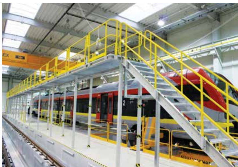
Lodz Agglomeration Railway depot
