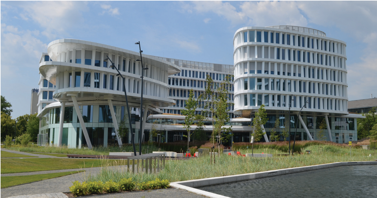
Fig. 1. Publicly accessible green area within the Wiśniowy Business Garden complex / Fot. J. Krajewska
