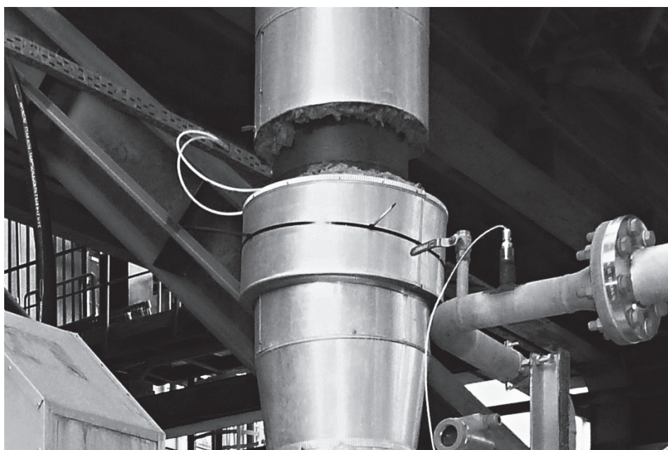
Fig. 8. View of the pressure grid installed in the pilot-scale plant
