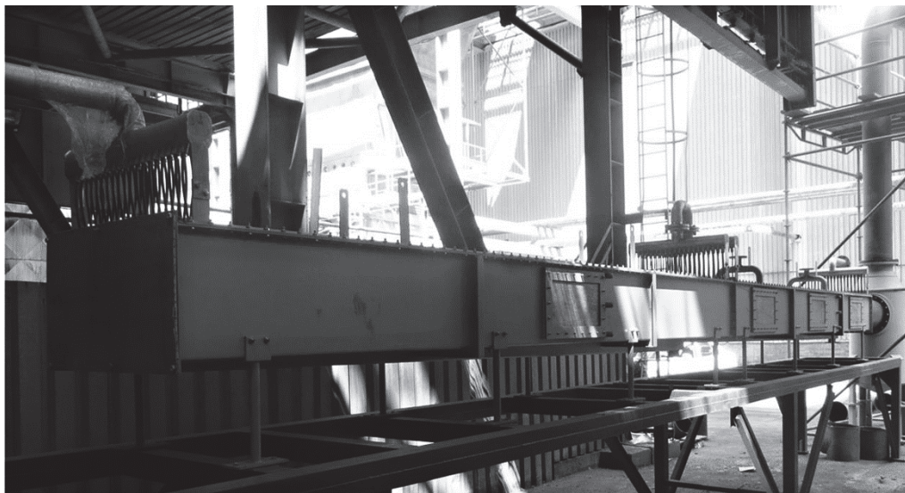
Fig. 3. View of the heat exchanger consisting of the condensing part and non-condensing part
