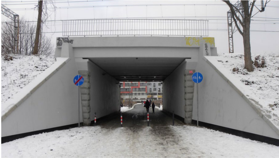
Fig. 3. Railway viaduct over Pawia Street. Own source
