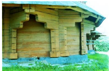
Fig. 16. The architectural enrichment of the forms of the wooden structures of the Orthodox church are often the protruding beams of the walls supporting the roofs - their forms vary depending on the local building traditions. Source: photo author
