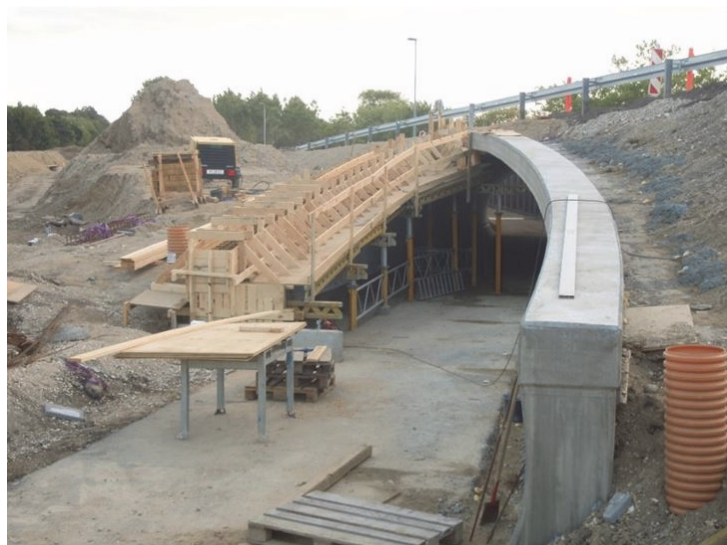
Figure 11. The formwork was made with accuracy – not an easy job
