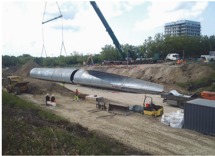
Figure 8. MultiPlate structure has been split into two parts – ready for lifting
