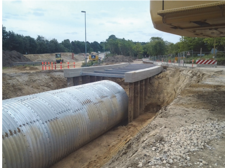
Figure 10. MultiPlate structure is placed between the sheet piling walls
