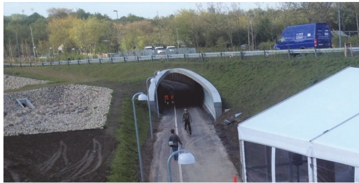
Figure 13. The MultiPlate structure is finished and the pedestrians use it every day
