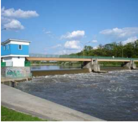
Fig. 3. Weir Opatowice – view from right bank
