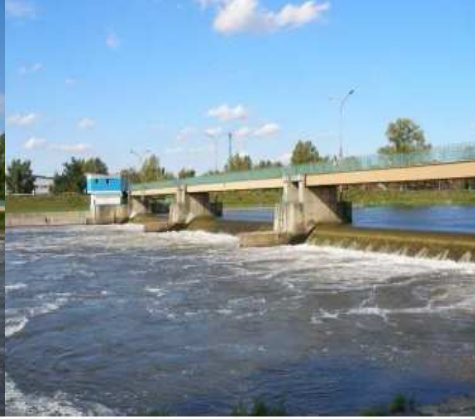
Fig. 4. Weir Opatowice – view from left bank
