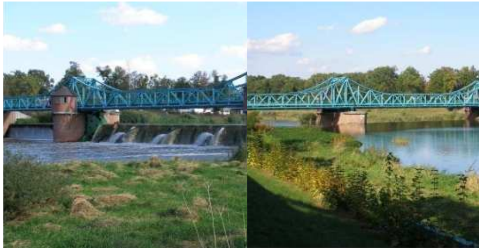
Fig. 1. Weir Bartoszowice from downstream side – view from left bank
