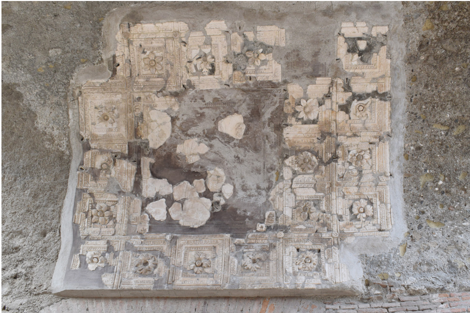
Fig. 4 Stucco Fragments repositioned on the barrel vault's inner surface on Maiuri's project. (Photo Credit: ISCR-Matera students)
