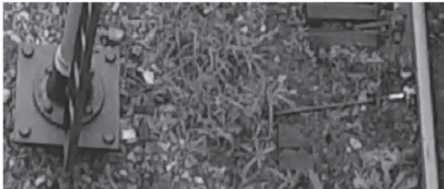
Fig. 4. Return wire of the shunt signal [own study]
