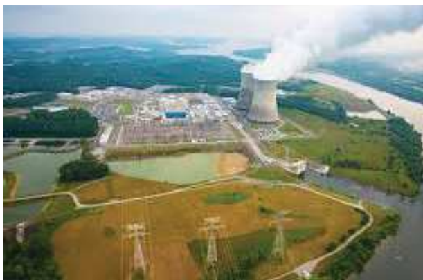
Fot. 1. Elektrownia jądrowa Watts Bar (Tennessee Valley Authority) Phot. 1. Watts Bar Nuclear Power Plant (Tennessee Valley Authority)
