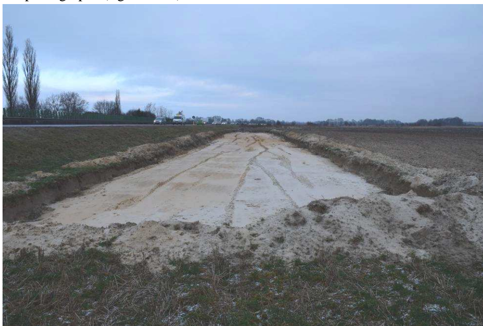
Fig. 3. View of the archaeological site at the stage of preparing the road construction
